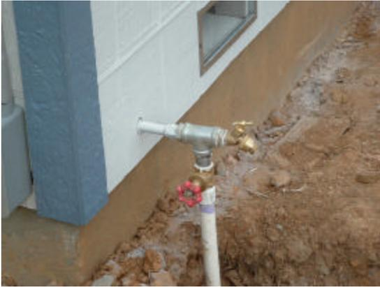
Metallic water pipes must be bonded to the home chassis.
