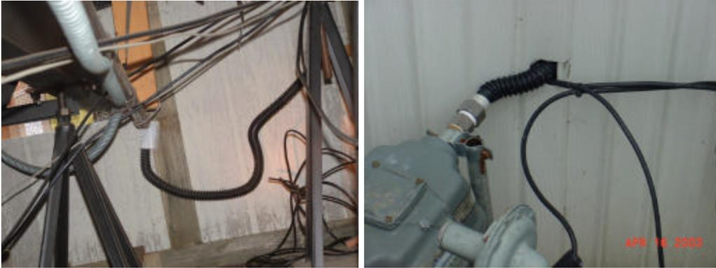
The gas pipe must be bonded to the chassis
