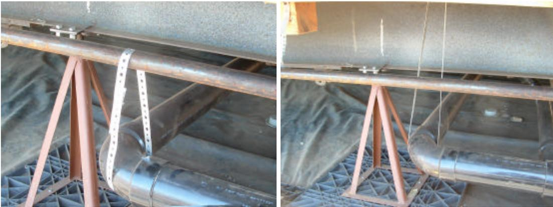
A combo fitting is a correct way to connect a second line to the system. Note the long sweep 90 degree connection.
