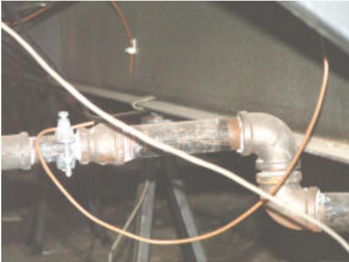
This factory installed water filter had loose fittings and leaked profusely.
