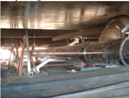
The level shows the correct fall of 2% slope towards the outlet to the right.
