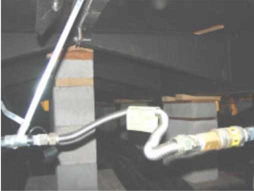
This cross over flex was found damaged and had to be replaced.
