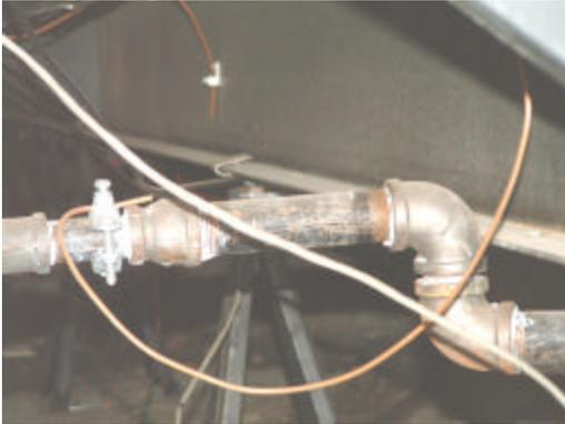
The gas pipe should be solidly attached to the home or framing where it stubs out.
