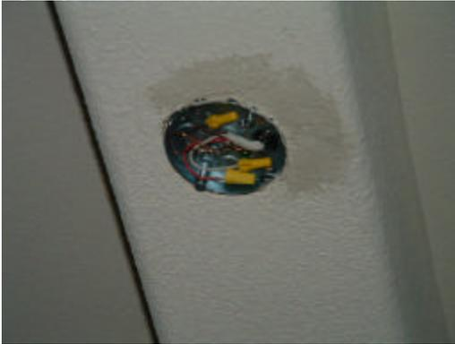
This electric crossover is unsafe. It should be sealed into the floor system, protected with nail plates at the joist notches and the connectors fastened to plan to the joists.
