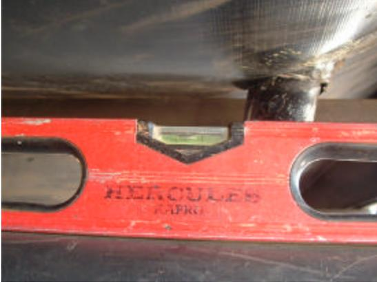
Measuring from the sewer pipe to the chassis or floor is a good way to set the straps for correct slope. For 2% slope, lower the pipe 1" every 4'.
