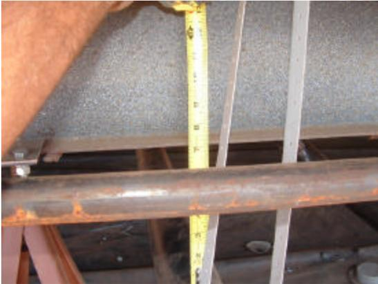
This section of pipes runs uphill for a section and must be re worked.
