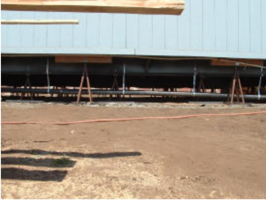
Straps must support sewer lines every 4'. Some inspectors require protecting the pipe with duct tape if using metal straps.
