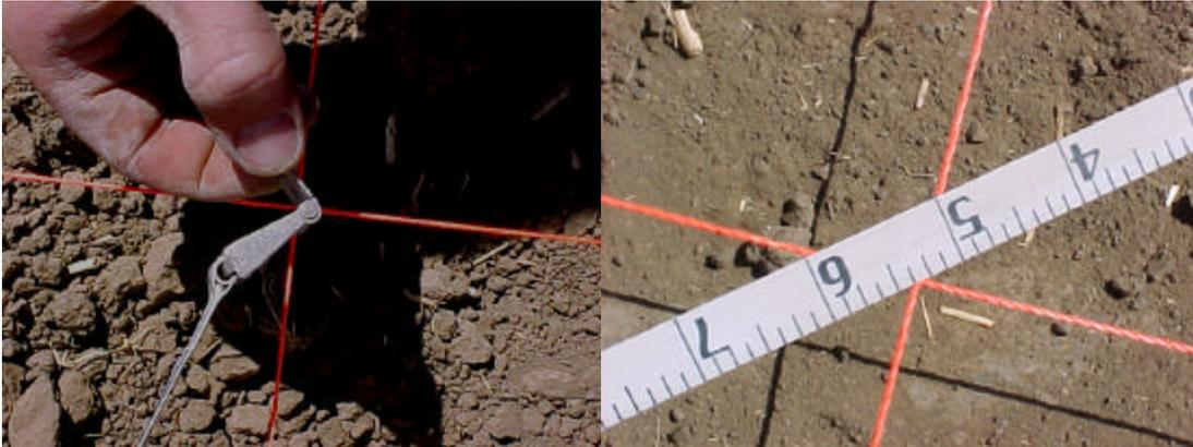
The screw inside is used for the forming, the center is the actual footprint and the outer is used to place the plate. By using offset string lines, the string can remain untouched and straight.
