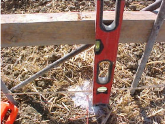
Measure from one batter board pin on the same wall side to set another batter board pin if a hub is lost.
