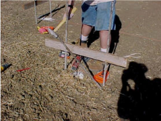
Measure from the layout hubs and transfer the offset from the tape measure to the batter board.
