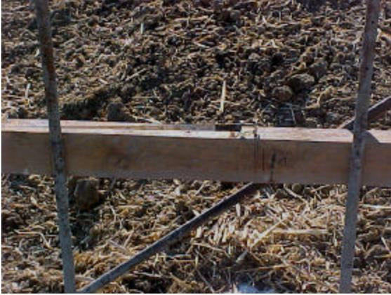
After the batter boards are all set and pinned, string line across all the boards to create a string around the largest dimensions of the home, then measure diagonals and perfect the batter board pins as needed by racking one pair fore and aft in equal amounts. When finished, the pins should measure the same as the home dimensions and the diagonals must be within 1/8".
