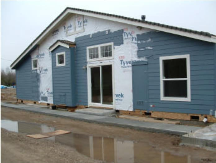
Using your eye or a string stretched across the sections. Ensure that the plank layout is reasonably true from section to section. This section is off and must be stripped and replaced.
