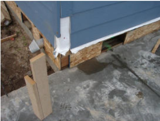
Next water proof the foundation framing or blocking with roof paper or house wrap, tucking the paper under the upper layer. Once the paper is finished, the trim can be fit and shimmed to plumb.
