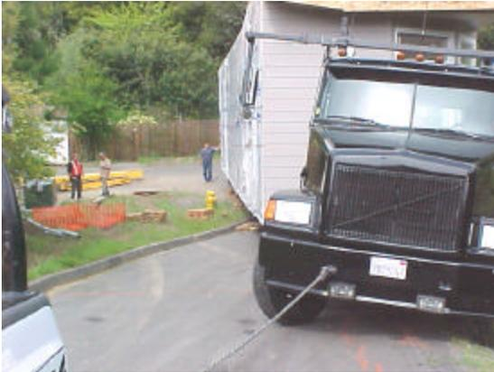
This home foundation was left open at the far end so two of three sections can be backed into the foundation instead of rolled over. This method creates additional cost in foundation work but saves on rolling and placement cost. I decide based on which resource has more time available, foundation crew or set crew.
