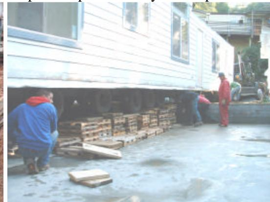
The Mobile Lift machine is used to pick up the unit and walk it around a turn in short lifts. It can lean from side to side as needed. It is a fine safety tool to lift the unit and support it while axles are removed and roller beams are installed. On smaller homes, the unit can lift the hitch end walk the entire home around. Care must be taken to not cause
